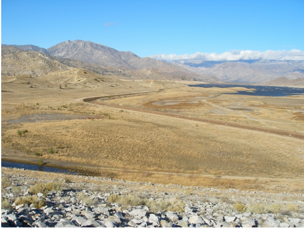
Figure 4. Upstream Portions of the Borel Canal Currently Visible due to Drought-Induced Low Water Conditions in Isabella Lake.
